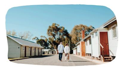
The buildings of Block 19 are in their original state. Bonegilla's army beginnings meant that accommodation was severe. The buildings were mostly standard army-type huts, usually unlined timber-framed huts with corrugated iron cladding and lowpitched, gabled roofs. Like the other blocks, Block 19 was self-contained with its communal kitchen, eating place and ablutions.
